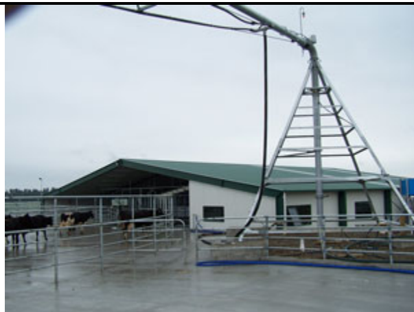
Parlor with Center Pivot System
